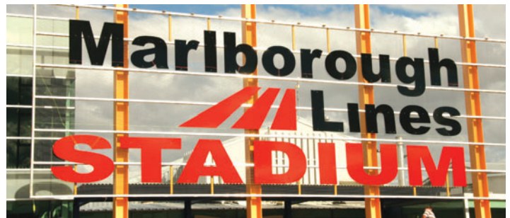
Marlborough Lines Stadium 2000
